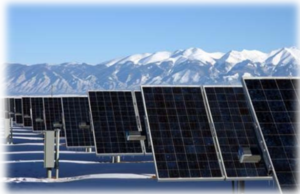
Solar Photovoltaic (PV)
