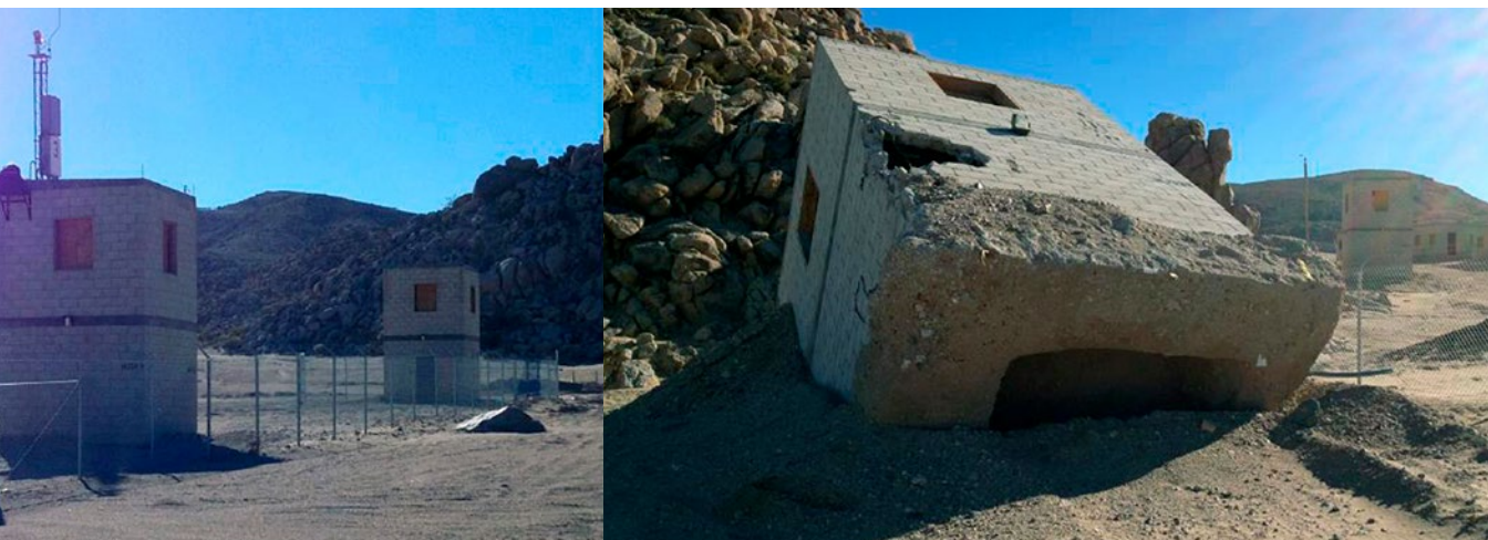
Guard towers at an Army training area in the Southwestern United States (left); the same type of guard tower, toppled and severely damaged by flash flooding from an extreme precipitation event at this training area (right). U.S. Government work.
